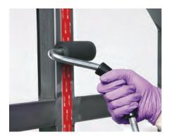
**STEP 3:** Apply pressure with a J-roller to at least 15 psi (100 kPa). This will help develop high-strength adhesion and bonding. Bond strength will increase after application.
